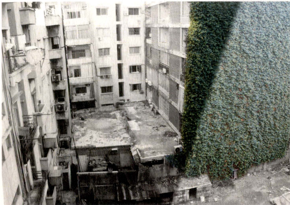
East View Overlooking The Transformers
