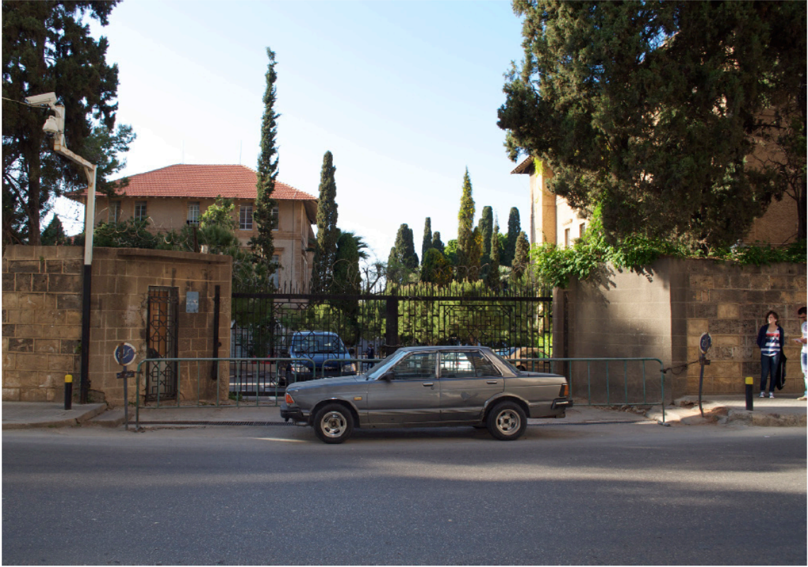
Picture 5: AUB wall fence on Bliss Street
