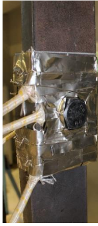
Figure. 4. Bolted lap joint wrapped in stainless steel foils
