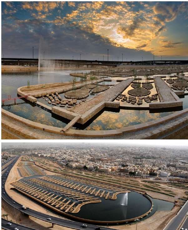
Figure 7. Bioremediation water treatment system in Wadi Hanifah, Riyadh, Saudi Arabia (the structure of biocells and the aerial photo of the bioremediation system). Source: Image courtesy of Arriyadh Development Authority and Google Earth, 2013.
