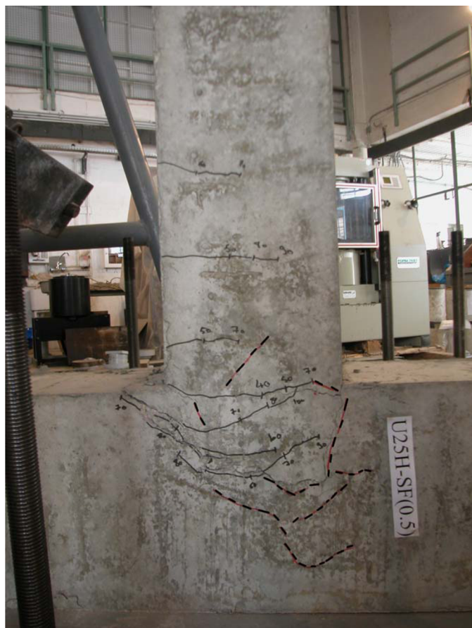
Fig. 6. Typical cracking pattern of the HSC beam-column specimen with 25-mm beam bars and 0.5% steel fibers; cracks shown in dotted lines happened after the specimen reached the maximum load and prior to halting the test (reprinted from Hamad and Abou Haidar 2011, © ASCE)
