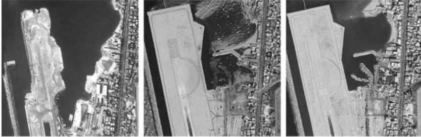
Figure 17. Evolution of Al-Hadi Port throughout the years Part labels (starting from left to right): a. Before the establishment of the Port- 1998, Source: Army Directorate b. The port in 2004, Source: Google Earth c. The port with a capacity of 336 boats in 2017, Source: Google Earth.
